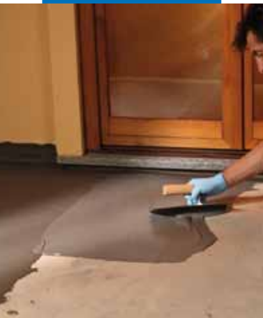
Waterproofing of terraces by trowel
