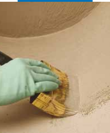
Waterproofing of details by brush
