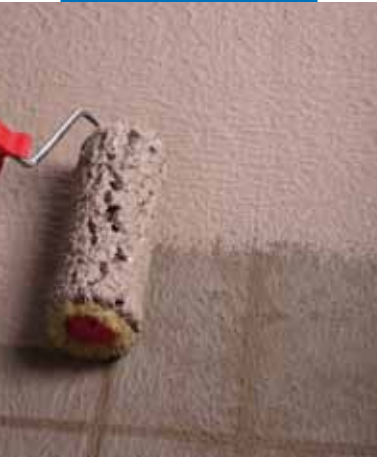
Waterproofing of details by roller
